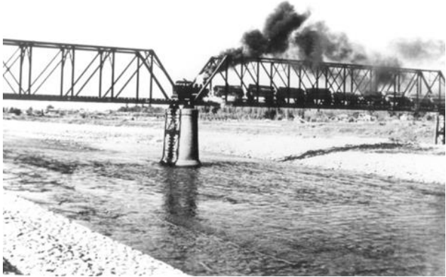
Diesel locomotive pulling railway cars with cedar logs across Nahari River in 1949
