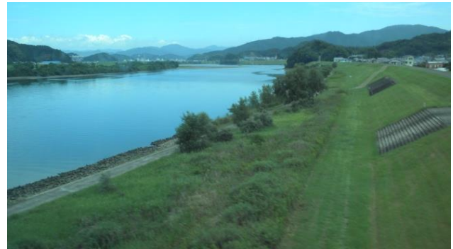
Protected levees along the Shimanto River
