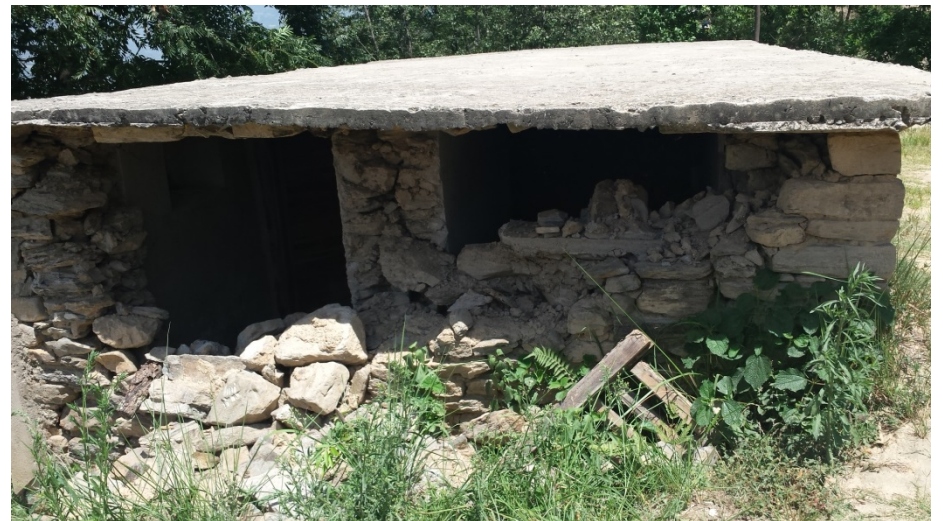
Crushed School Toilet (Thansing village)
