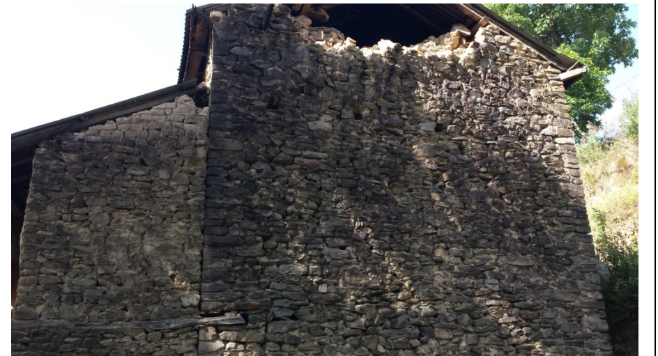
Damaged House of Tulasi and family (staying with relatives). Given Rs.800 to neighbor Jayaram Adhikari(Local Volunteer coordinating our effort) to give to Tulasi
