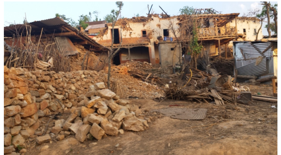
This village (Adhabaat) was one of the worst hit. One person died in the two-story building above. We provided some cash help to the family
